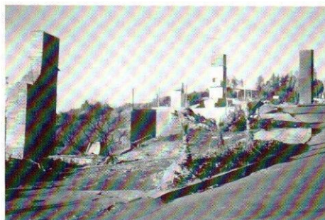
On November 6, 1961, a brush fire driven by 50 to 70 miles per hour Santa Ana winds in 100° F, 6% relative humidity weather burned from the top of Beverly Glen Boulevard south and west to the ocean. By nightfall, 560 homes had been burned.
